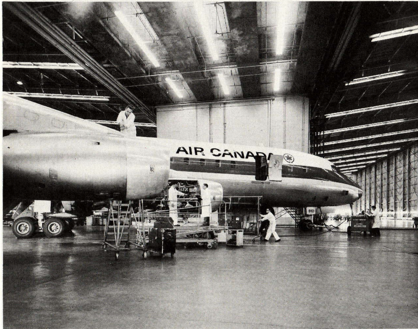
The Line Maintenance Hangar measures 487 feet by 235 feet with 50-foot high doors. It can accommodate either three DC-8 and five Vanguard aircraft or two DC-8s, four Vanguards and four Viscounts at one time. Maintenance checks are scheduled ahead of time and are performed around the clock.
